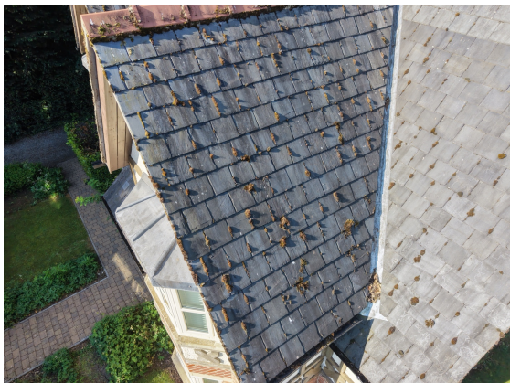
BEFORE · ROOF CONDITION
