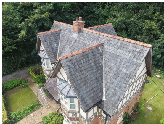
AFTER · COMPLETED PROJECT VIEW
